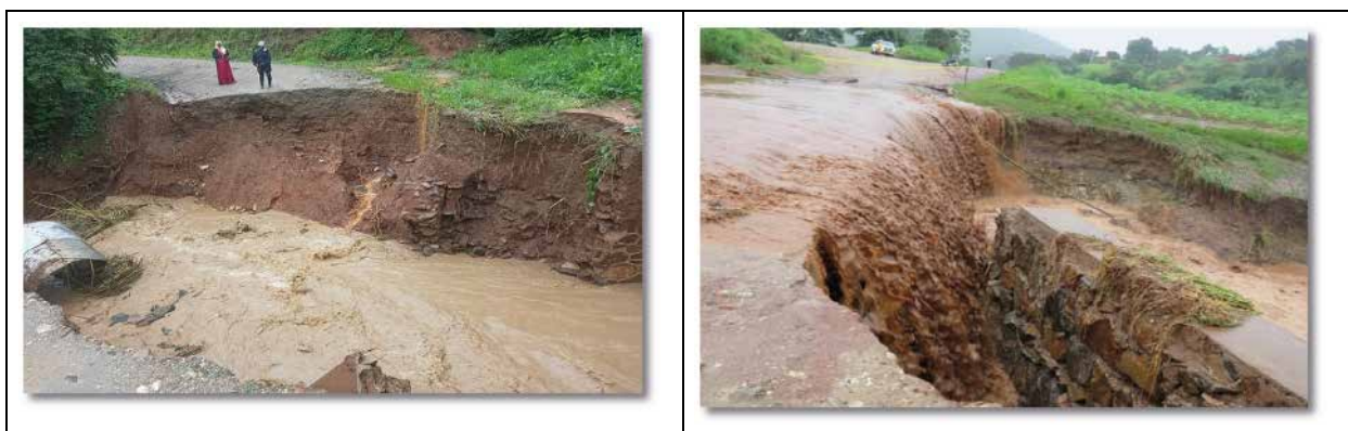
Figure 12: Nyapinda Bridge was damaged because of heavy rainfall that occurred on 22 nd and 23 rd February 2022 (Source: Nipashe Newspaper, 24 th February 2022).
